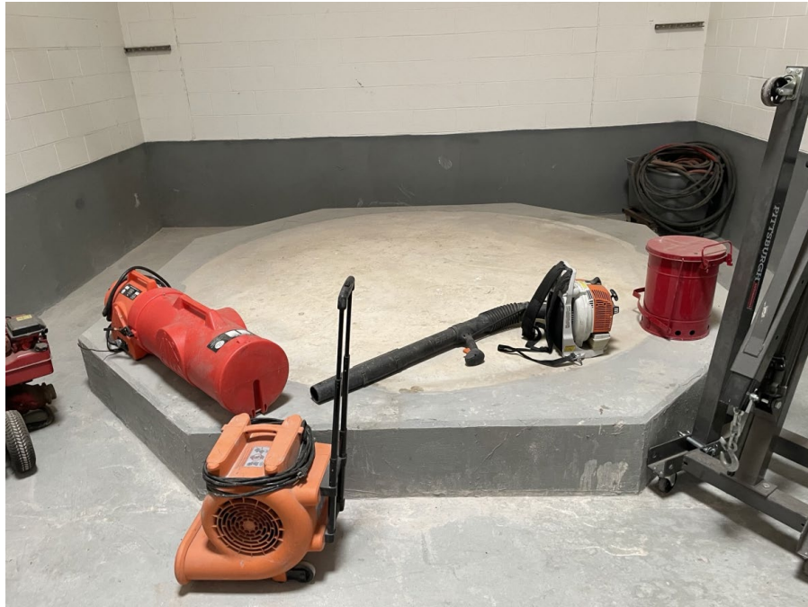
Existing room that will be converted into new electrical room.
