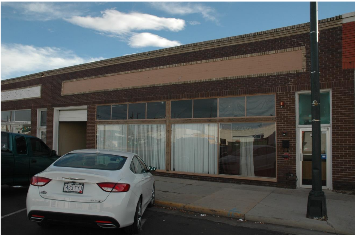
CD 1, Image 165, View to SE of west half of façade (east)
