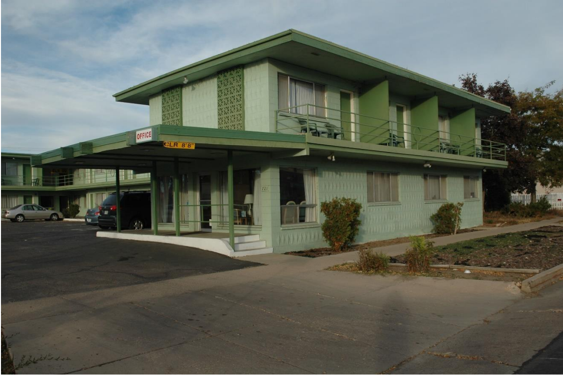
CD 1, Image 210, View to NE of south and west sides of the office
