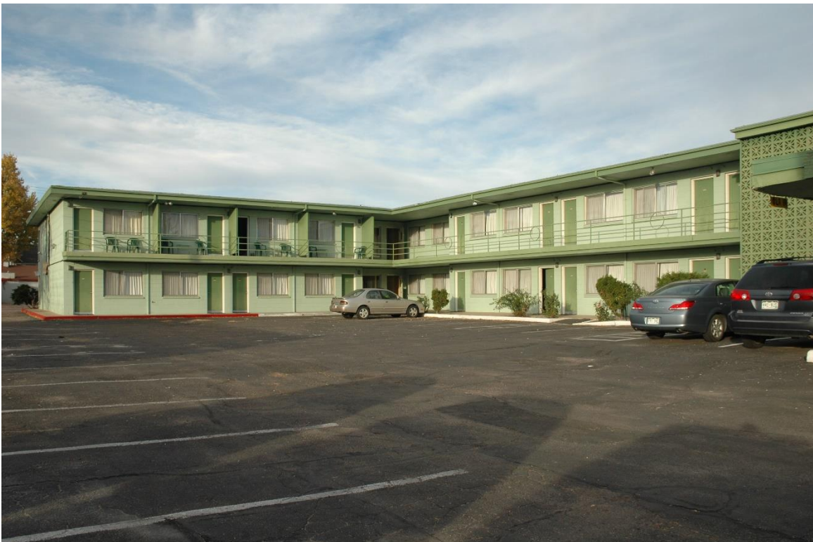
CD 1, Image 213, View to NNE of rooms facing onto parking lot
