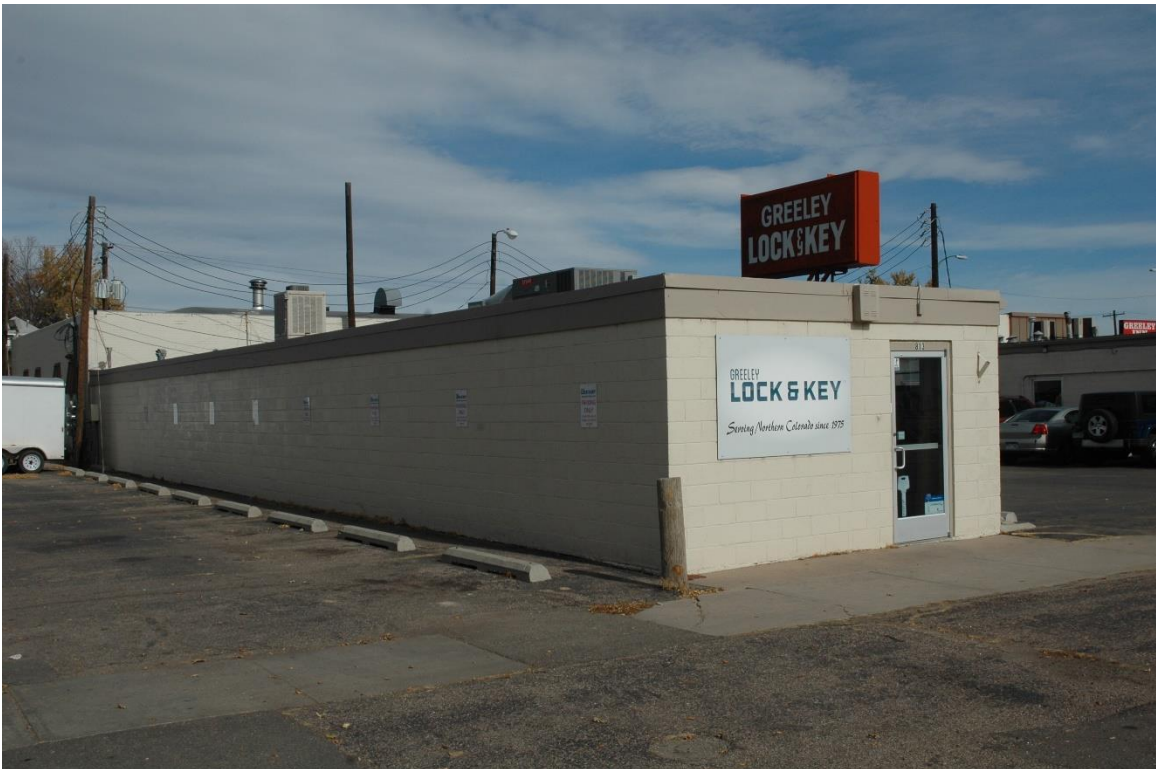
CD 1, Image 60, View to NE of façade (south) and west side
