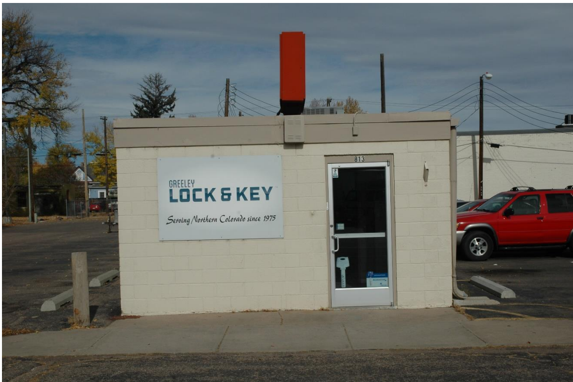
CD 1, Image 61, View to north of façade (south)
