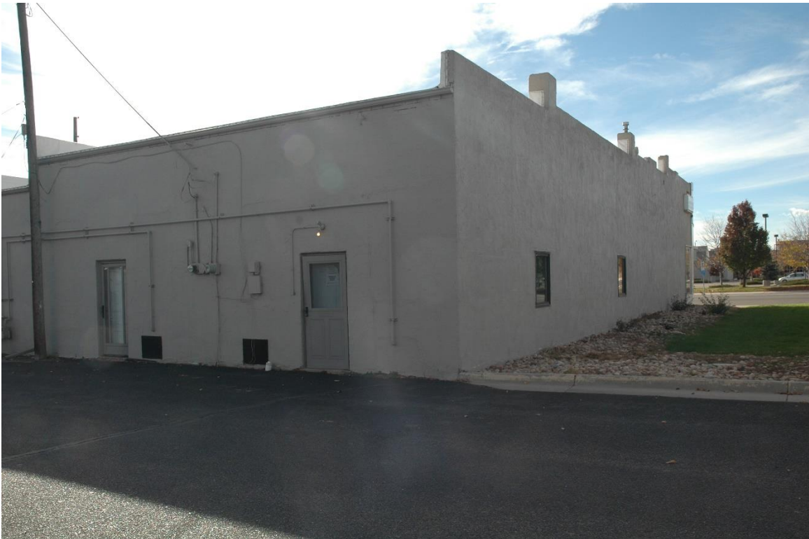
CD 1, Image 145, View to SW of rear (east) and north side
