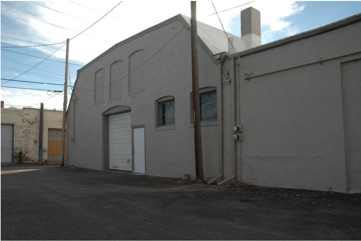
CD 1, Image 148, View to SW of rear (east)
