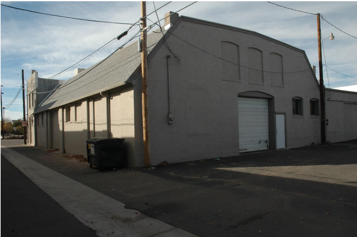
CD 1, Image 149, View to NW of rear (east) and south side
