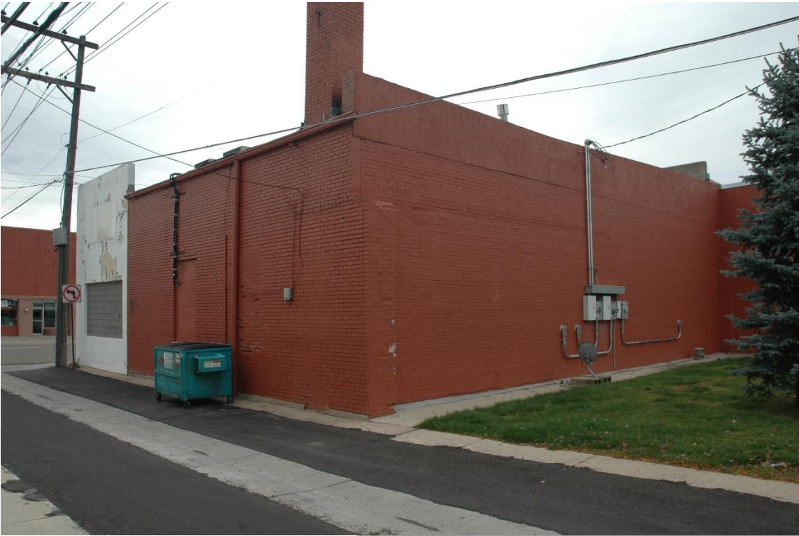
CD 1, Image 3, View to SE of rear SW corner
