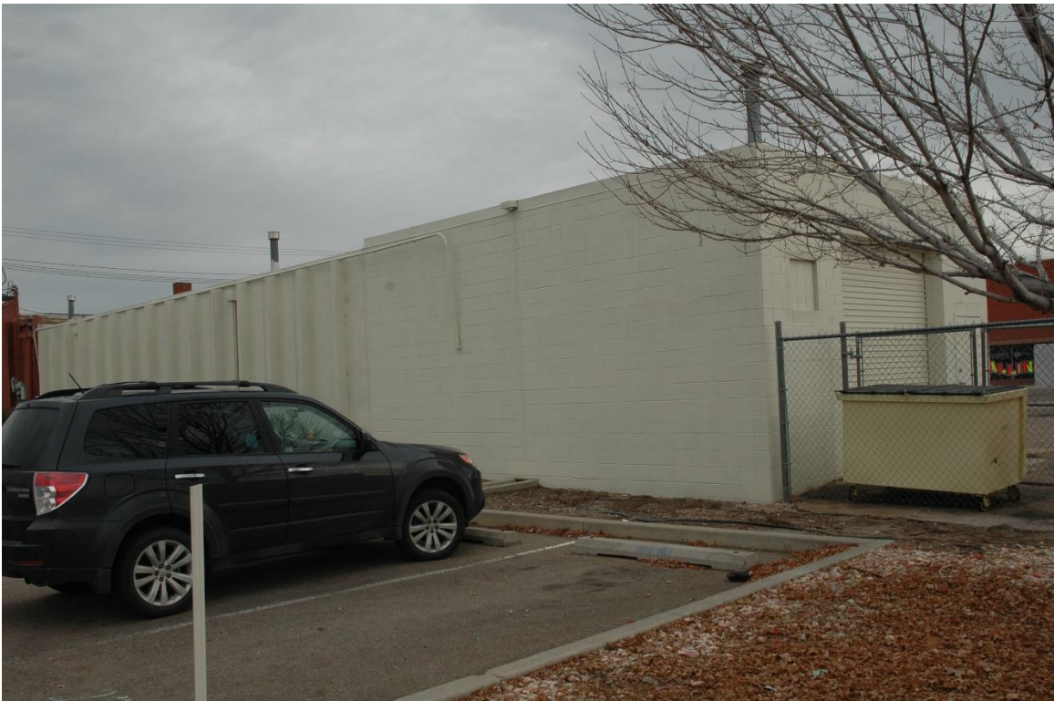
CD 1, Image 13, View to NE of rear (west)
