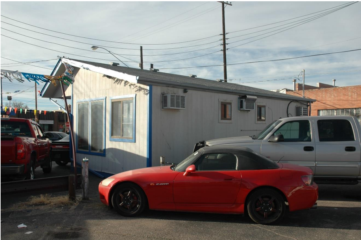
CD 1, Image 185, View to NW of rear (east) and south side
