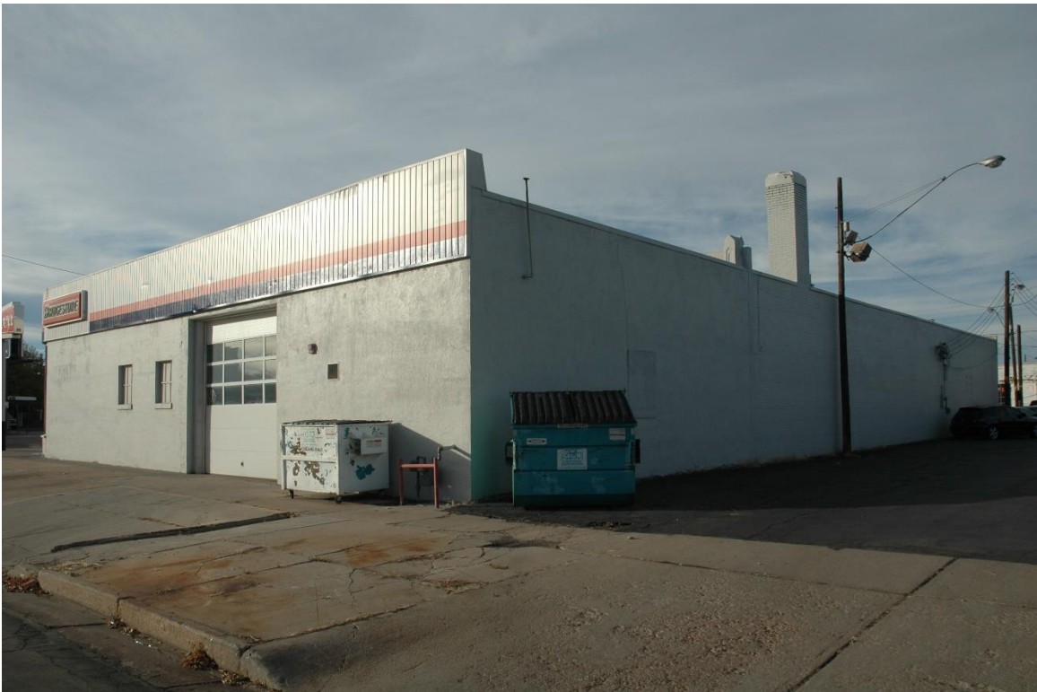
CD 1, Image 187, View to NW of rear (east) and south side
