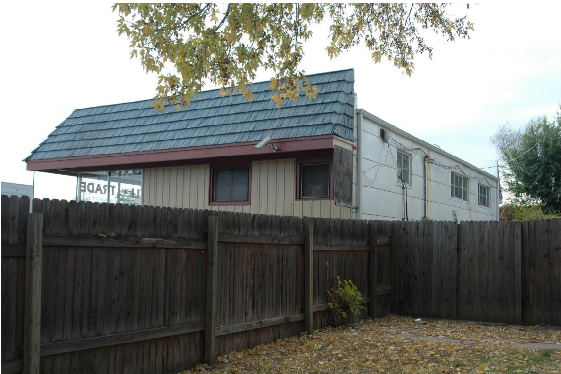
CD 1, Image 43, View to SE of rear (west) and north side
