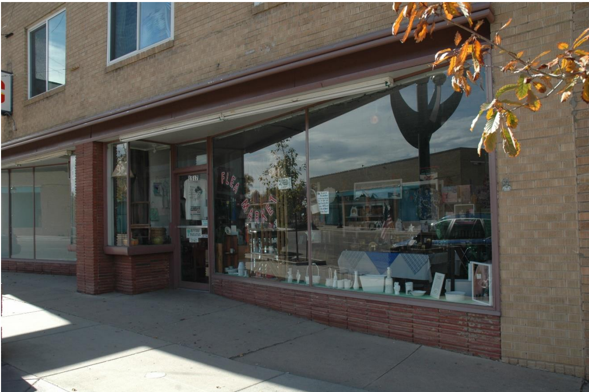
CD 1, Image 113, View to SW of lower façade (east)
