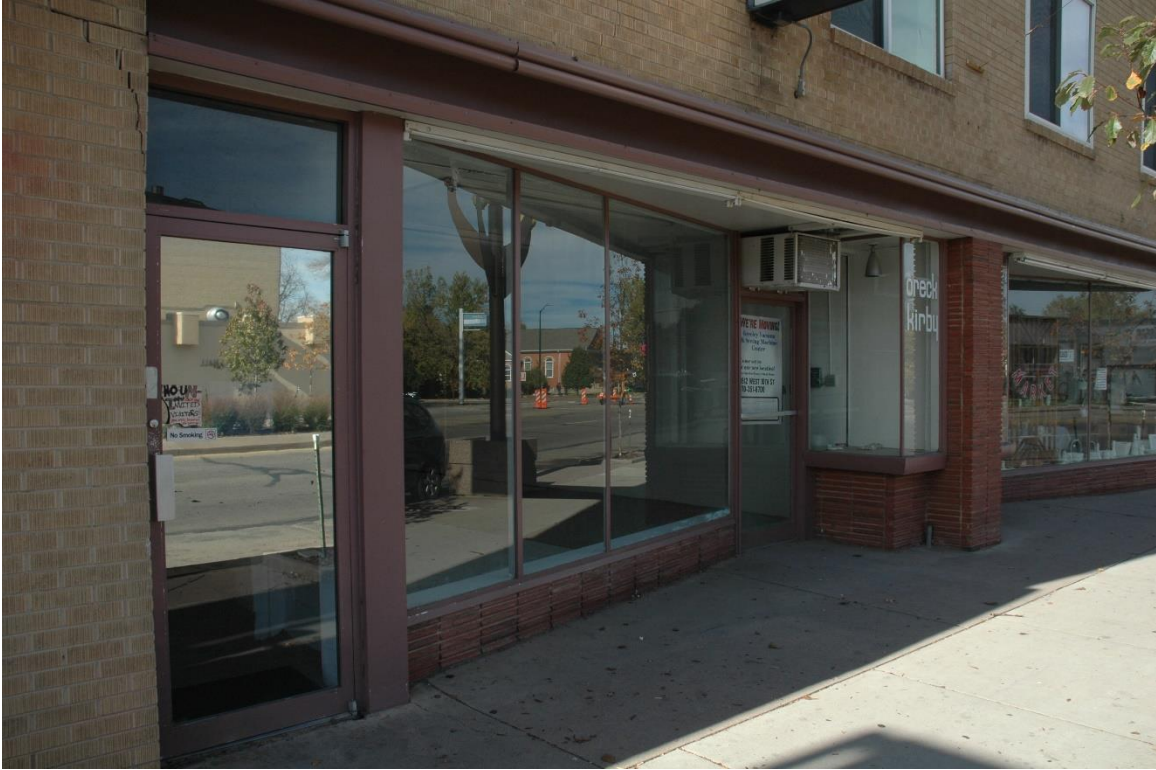
CD 1, Image 112, View to NW of lower façade (east)
