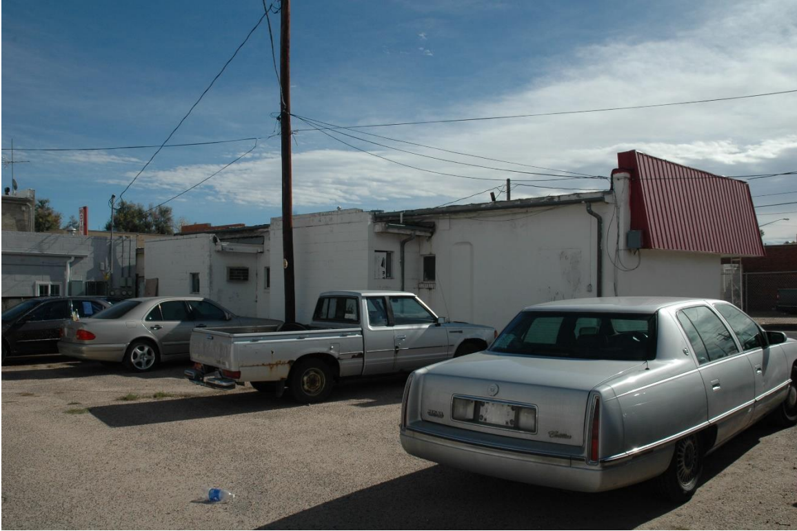
CD 1, Image 116, View to SE of north side and rear (west)
