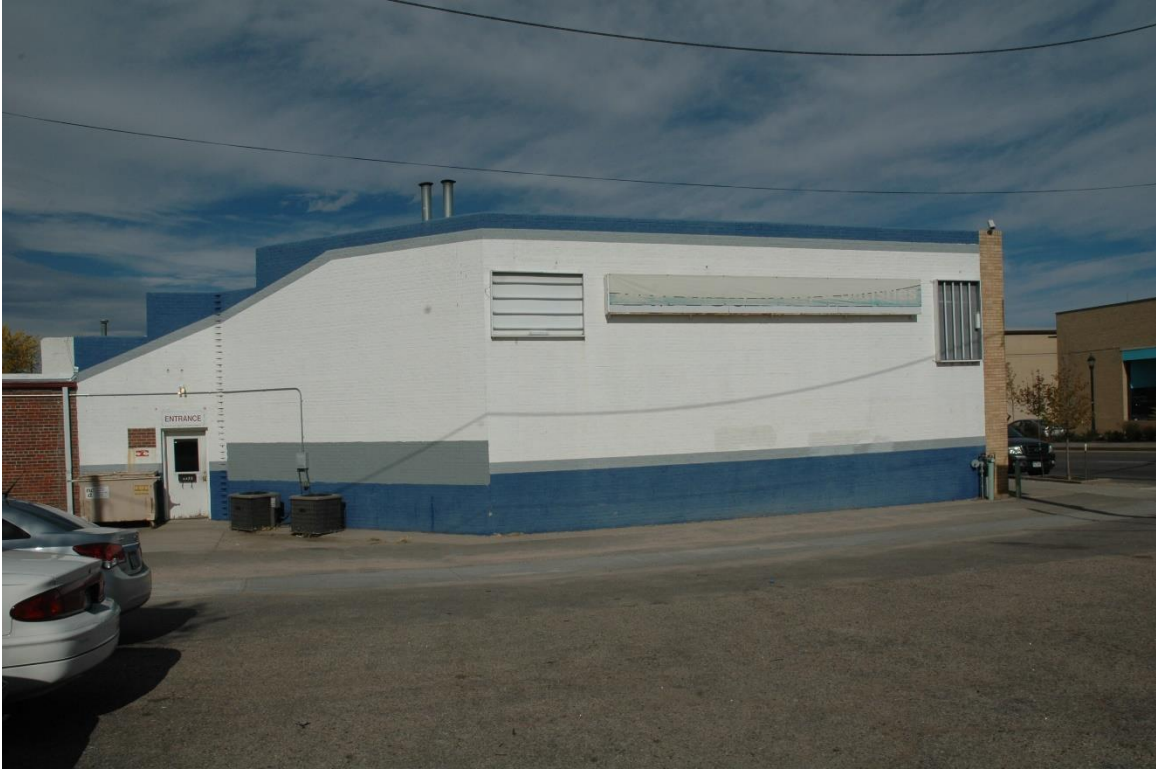
CD 1, Image 126, View to north of front portion of south side
