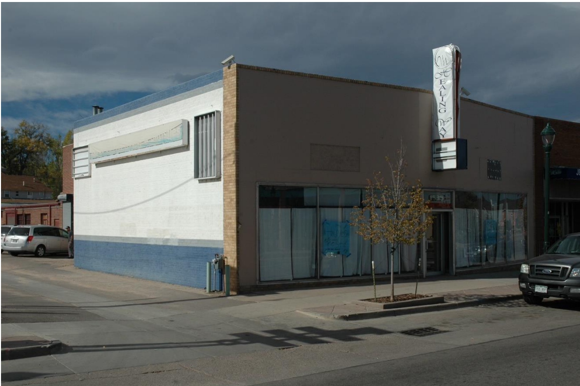
CD 1, Image 125 View to NW of façade (east) and front portion of south side
